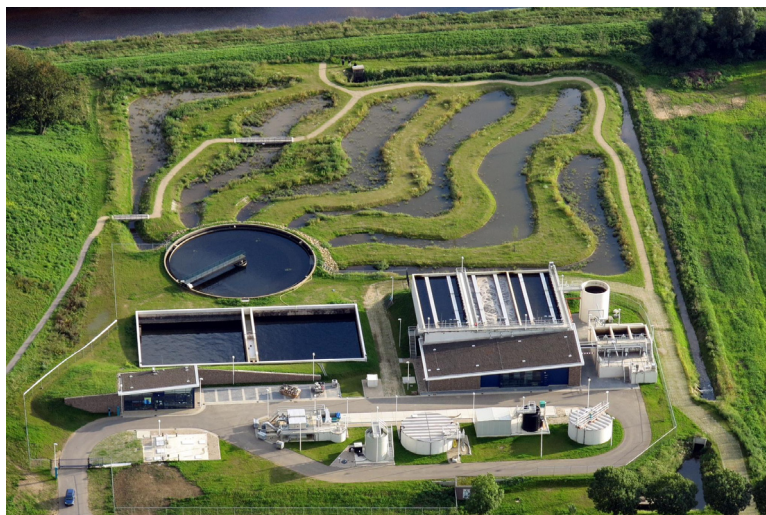
Fig. 1. Photograph of WWTP in Dinxperlo, the Netherlands. The Nereda® reactors are located on the right, attached to the building with the sloped roof. The sludge buffer and the sand filter are located to the right of the Nereda® reactors. The inlet works, including the influent buffer are located at the bottom. The old pre-existing aeration tank and clarifier on the left are now part of a public water garden (on the top).
