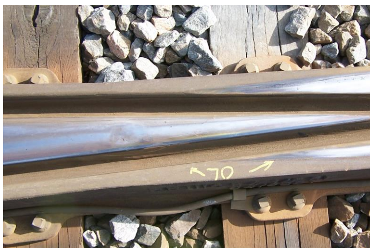
Figure 2.1. RCF damage at railway crossing
