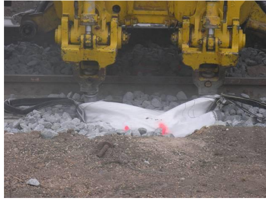
b. Field tests of tamping (ballast bag); figure reproduced from [41]
