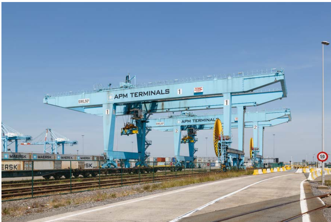
Figure 4.26: APMT Zeebrugge (Belgium) rail terminal with gantry crane (by CEphoto, Uwe Aranas is licenced under CC-BY-SA 3.0).
